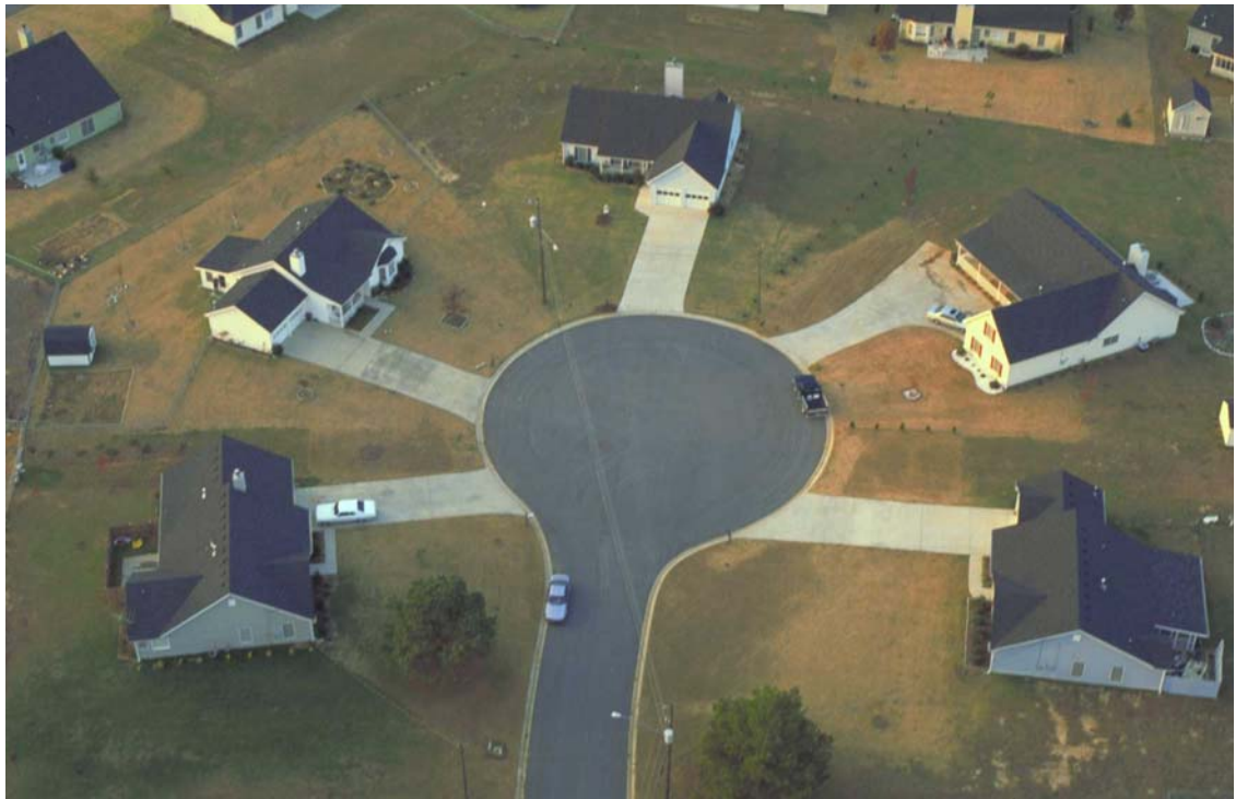
Figure 11: A Suburban Subdivision
