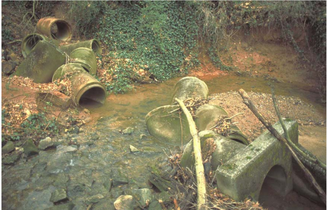
Figure 16: Destructive Potential of Development-Induced Stream Channel Enlargement
