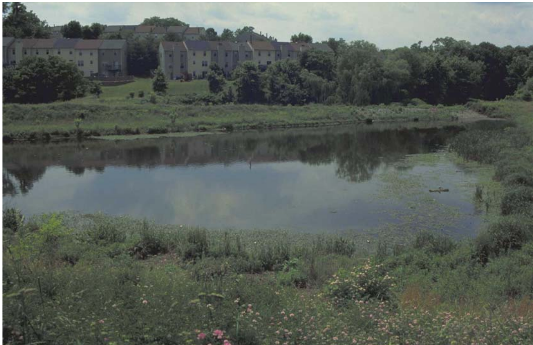
Figure 22: Stormwater Pond on Weaton Branch
