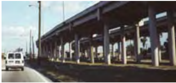
Typical trestle-type construction as seen on the early segment of the Selman Crosstown Expressway through downtown Tampa. Picture from Tampa Hillsborough County Expressway Authority.
