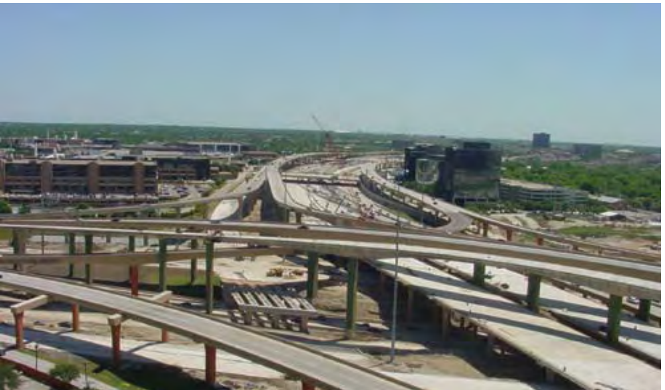
New interchange at I-635 and US-75 in northwest Dallas known as the High Five for its five levels of soaring ramps. Pictures from Texas DOT, Dallas District on Web site of Texas Freeway.
