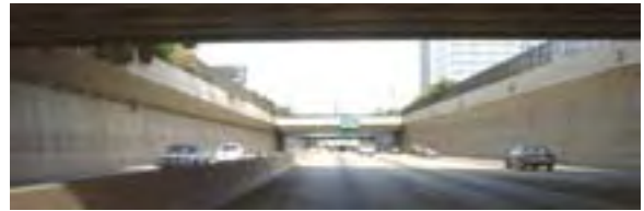
At two miles long, the Vine Street Expressway (I-676) is depressed below ground level in a walled trench and skirts the northern fringe of Philadelphia's central business district.
