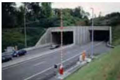
A tunnel under developed areas enabled a radial motorway, the A14, to be built west out of Paris. It was financed by a toll concession granted to SAPN (Societe des Auto-routes Paris-Normandie). With only 2x2 lanes, the tunnel toll is raised in peak periods to encourage some traffic to travel off-peak, maintaining free flow. Picture from SAPN.
