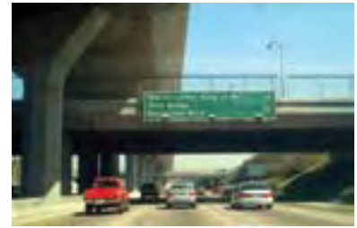
I-110 Transitway, just south of downtown Los Angeles is elevated above the cross bridges as well as the main lanes.
