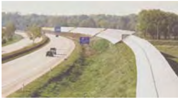
Sound berm on the A92 motorway near Freising in southern Germany is used to mount arrays of photovoltaics called Das Projekt PV-Soundless. Photo from solarintegration.de .
