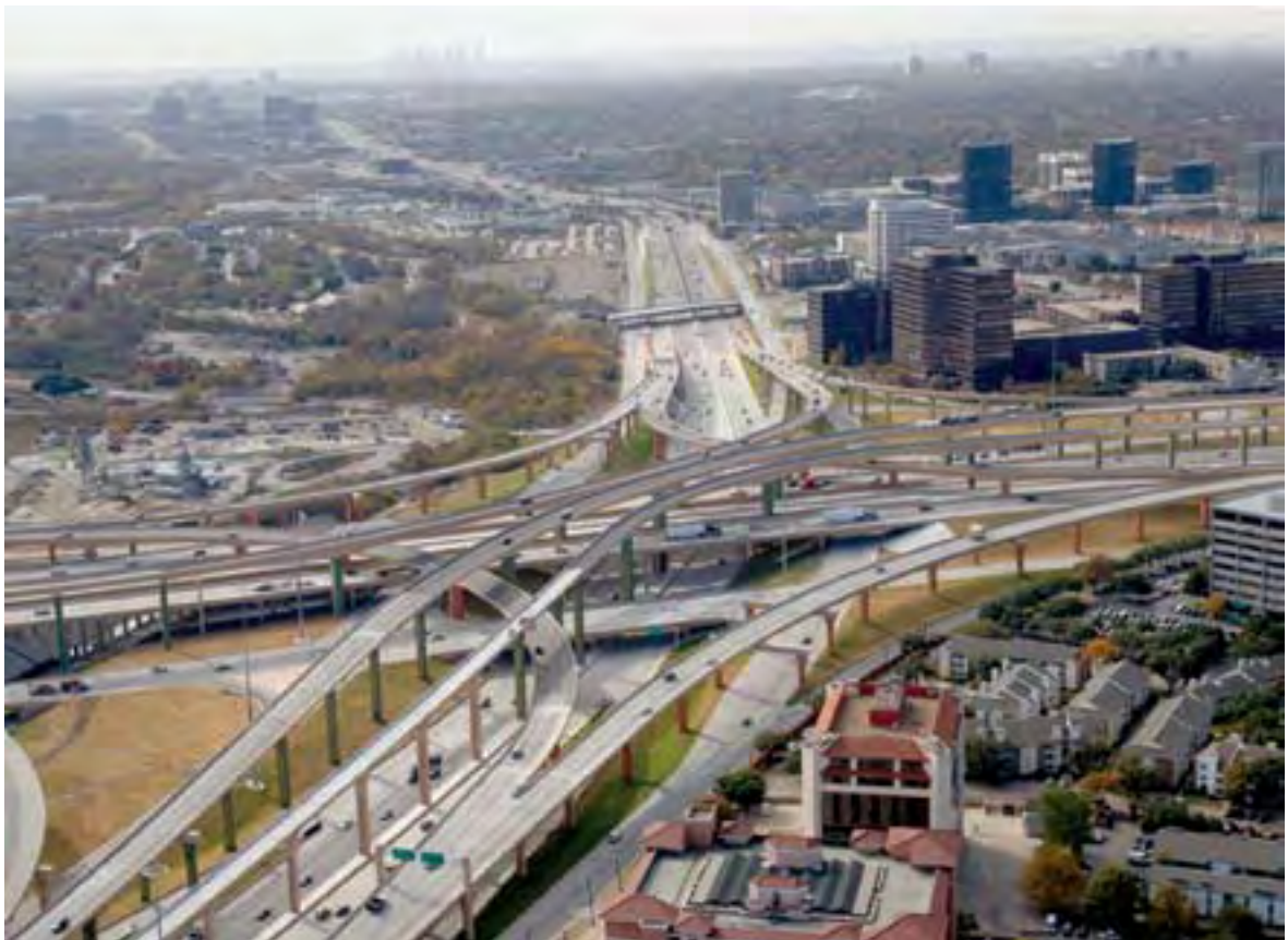
The "High Five" interchange, at the intersection of interstate 635 and US Highway 75 in Dallas. Photo by Kevin Brown.
