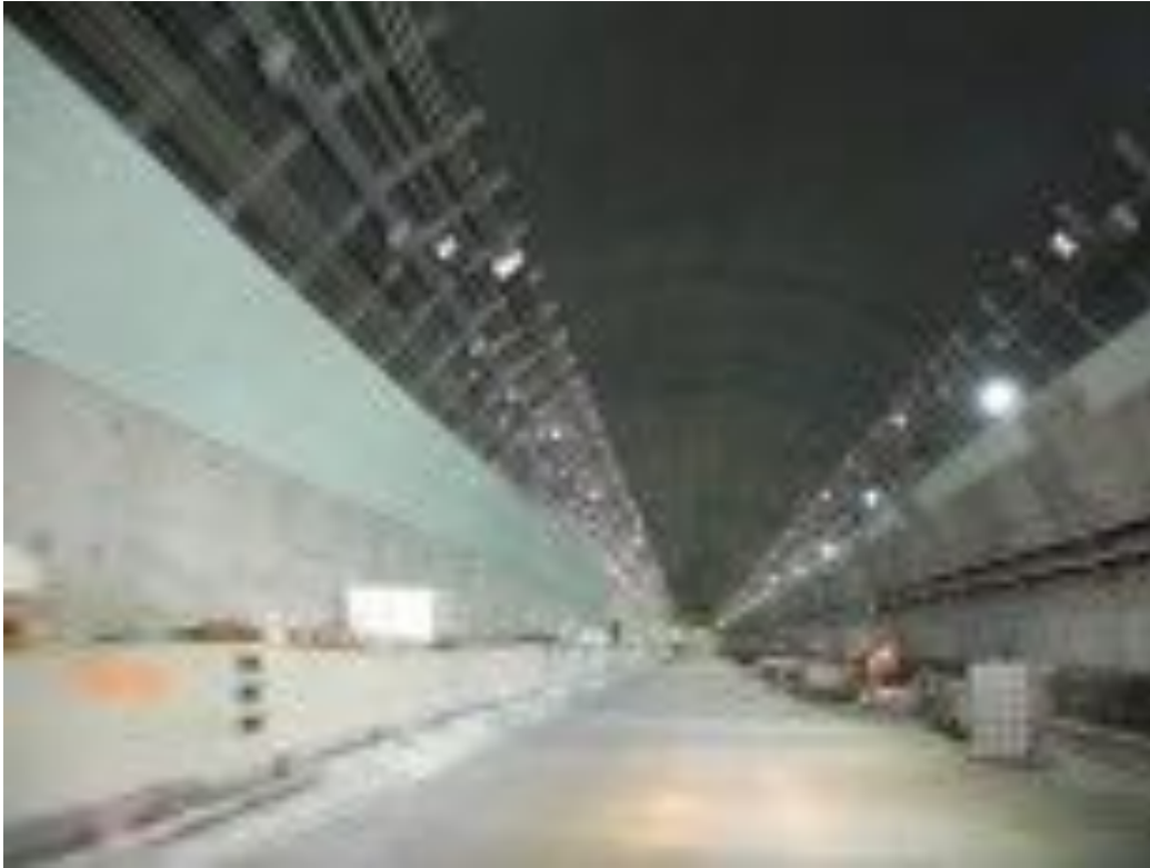
Figure 37: Port of Miami Tunnel
