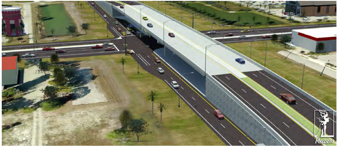
Figure 4: Typical Arterial Overpass
